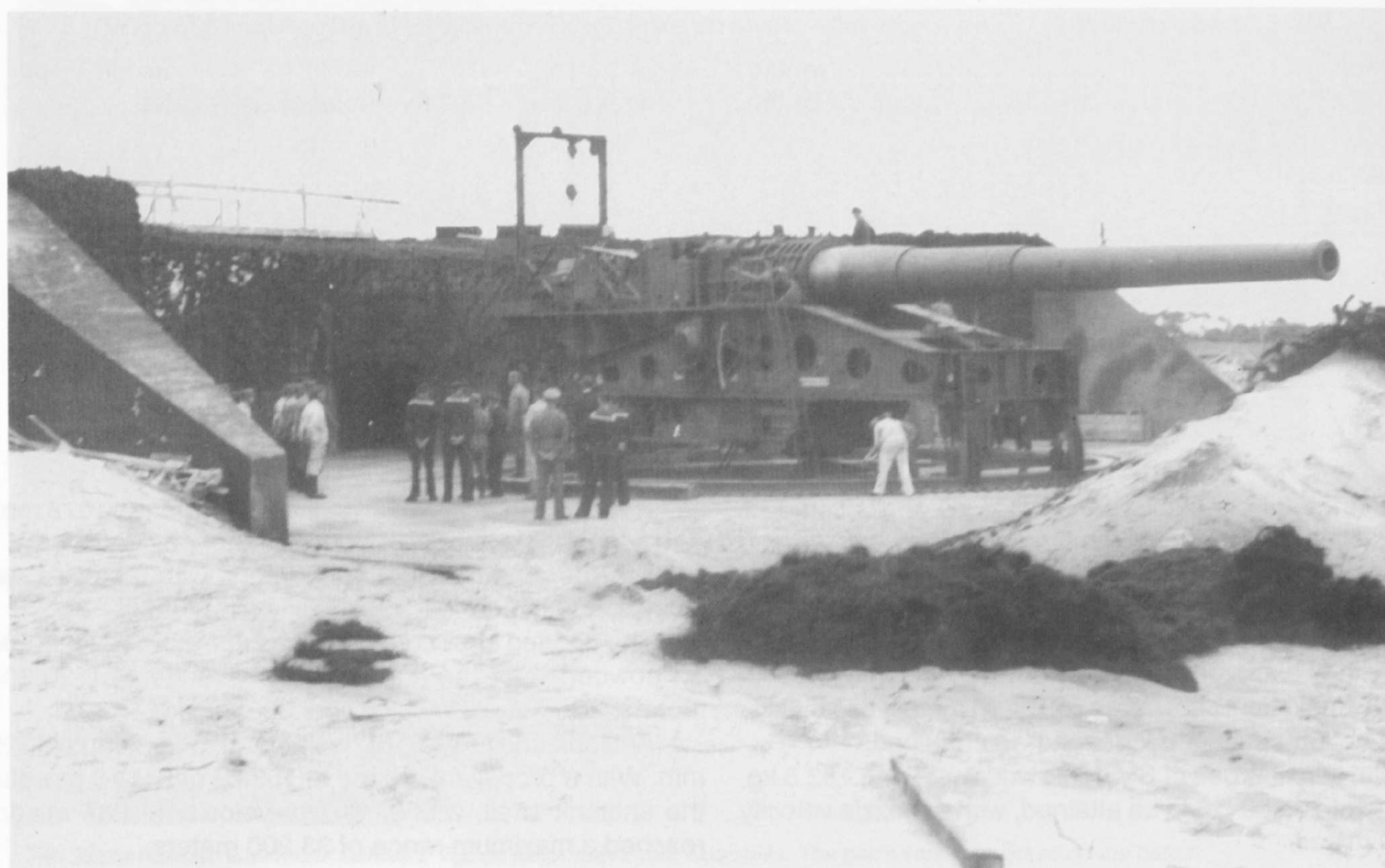
Below: The third gun is being installed in its bed.
