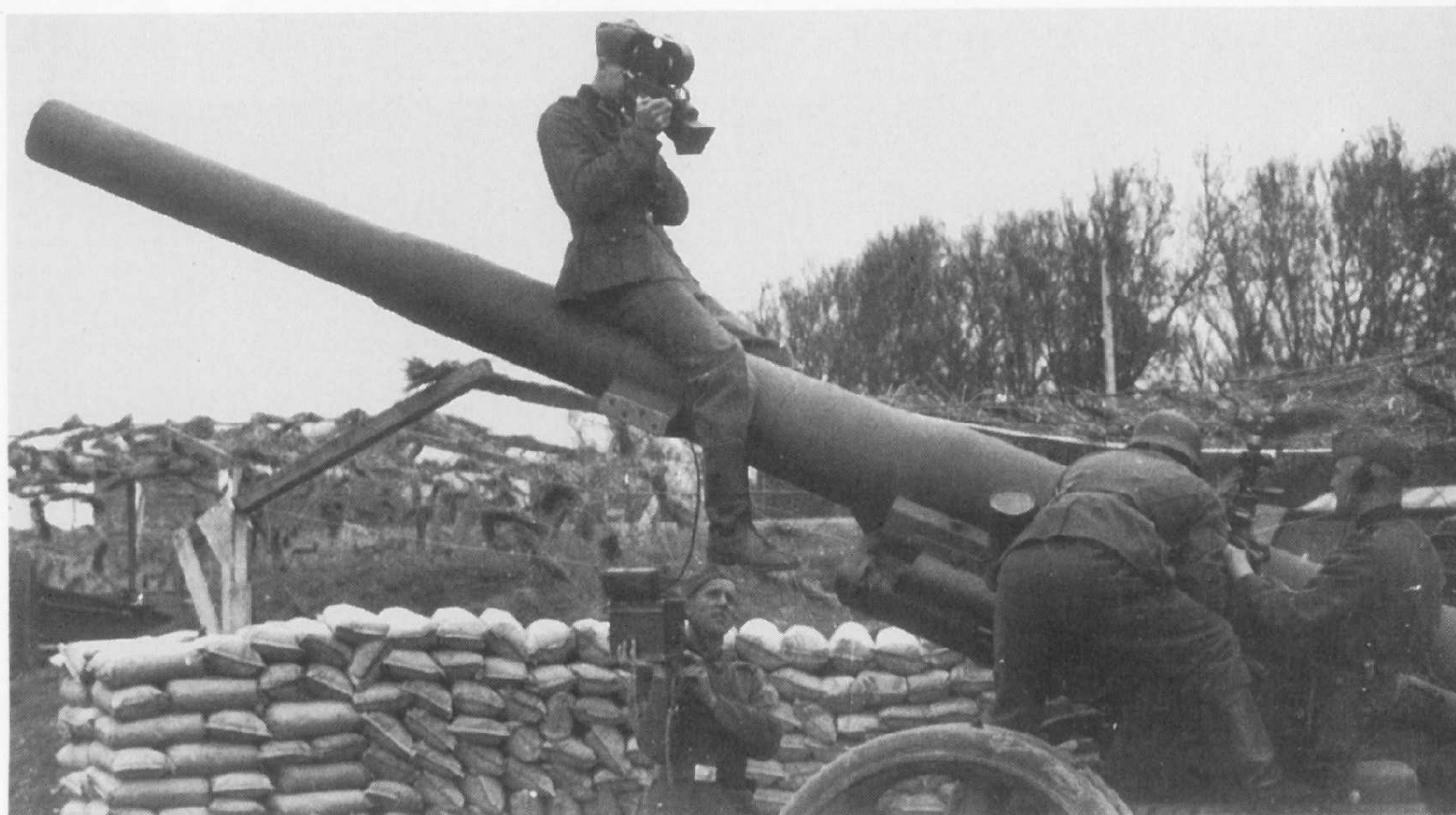
A war correspondent films the process of aiming a 15.5 cm Field Cannon 418 (f). The aiming gunner, at far right, receives the shot values from the command post through headphones. The elevation gunner, at his left, cranks the barrel to the ordered height. The aiming optics can be seen in front of the aiming gunner.
