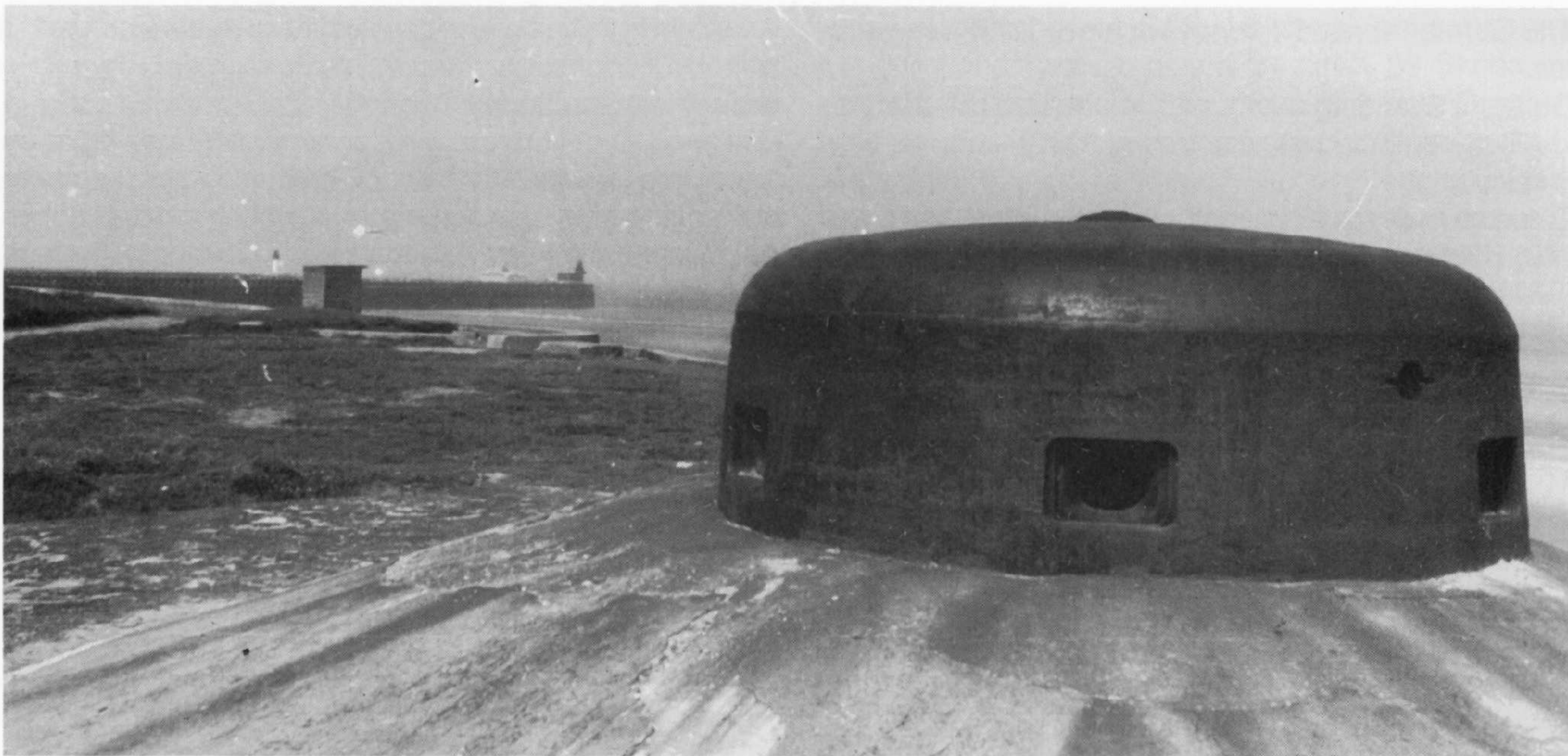
In the 6 Scharren turrets, two machine guns on Scharren Mount 34 could be set up, as well as a parabolic telescope with fivefold enlargement and 14-degree field of vision around 360 degrees. These armored turrets, manufactured by Krupp, proved themselves very well in the fighting on the Atlantic Wall and withstood even the heaviest fire. The picture shows a 6 Scharren Turret at the entrance to Calais harbor.
