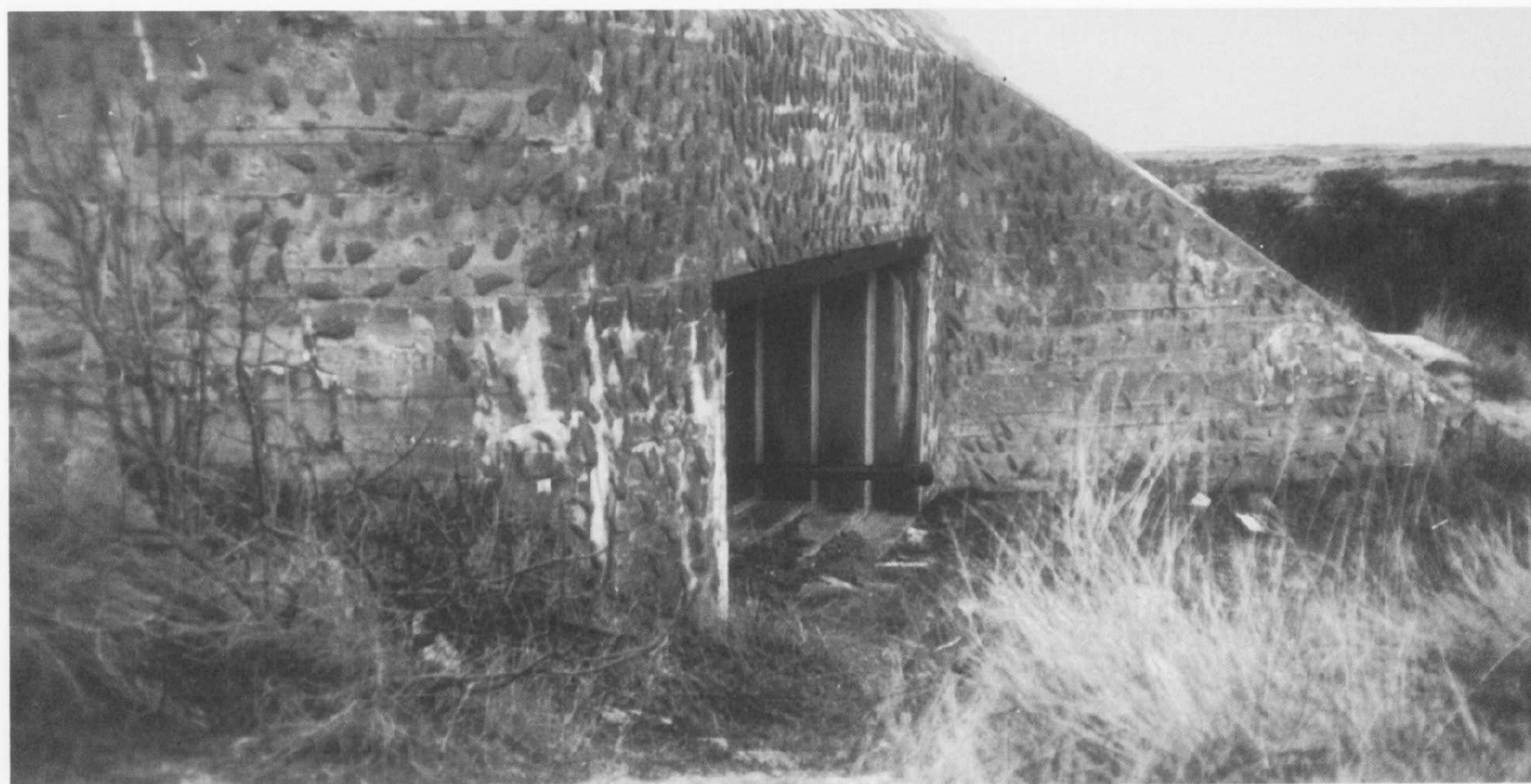
Left and below: The 5 cm KwK were often flanking, pointing along the shoreline. On the ocean side, the bunker and gun barrel were protected from enemy naval fire. The upper photo shows standard bunker 667, the lower one standard bunker 613.
