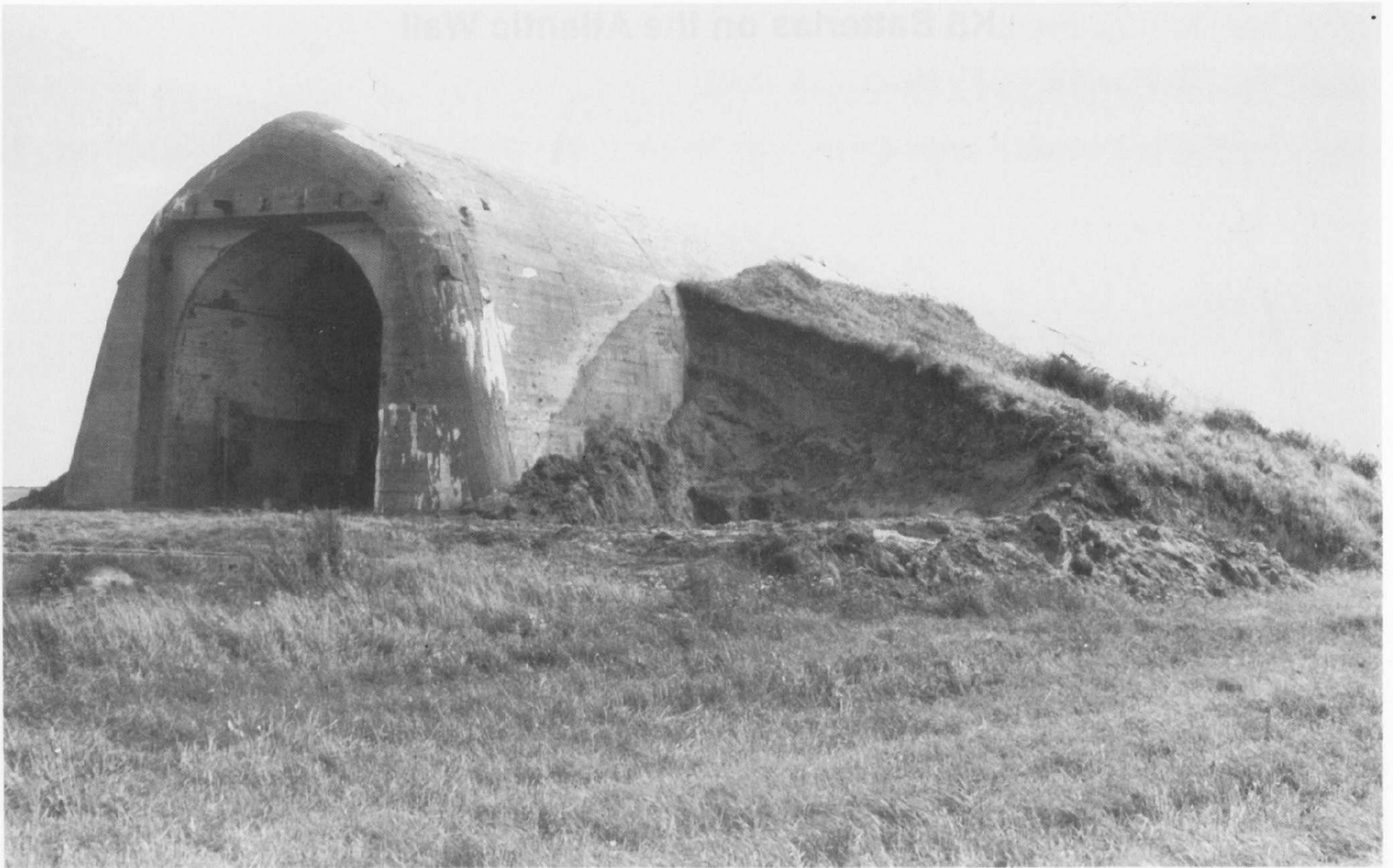
A domed bunker of Battery E 712, with soil banked against it. The arched form of the bunker's roof was meant to deflect striking shells off to the side.
